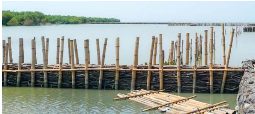
Fig. 4. Permeable bamboo wave screen at Demak, Indonesia [3]
